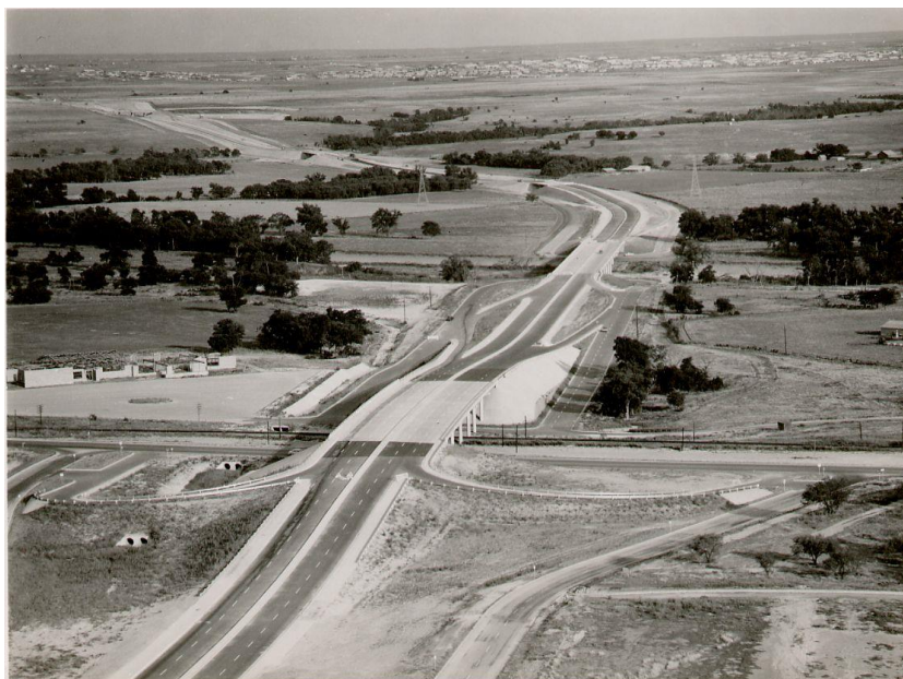
4597 Loop 217, Stove Foundry and Texas & Pacific RR
